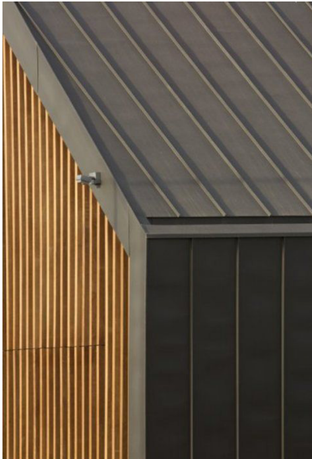
MATERIALITY DETAIL Zinc roof with timber cladding
